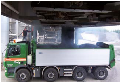
Asphalt and concrete mixing
